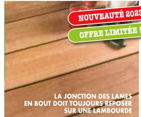
LA JONCTION DES LAMES EN BOUT DOIT TOUJOURS REPOSER SUR UNE LAMBOURDE
